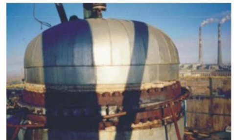
After 46" clamp intalled and sealed
